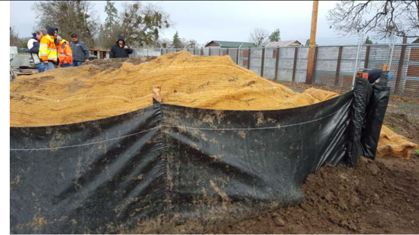
RVSS Erosion Prevention and Sediment Control Inspector Training
