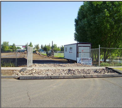
Source: City of Bend
